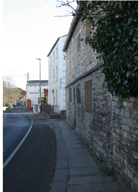
Looking down Main Street by the Grade II listed Malvern House. Note the width of the pavement.
