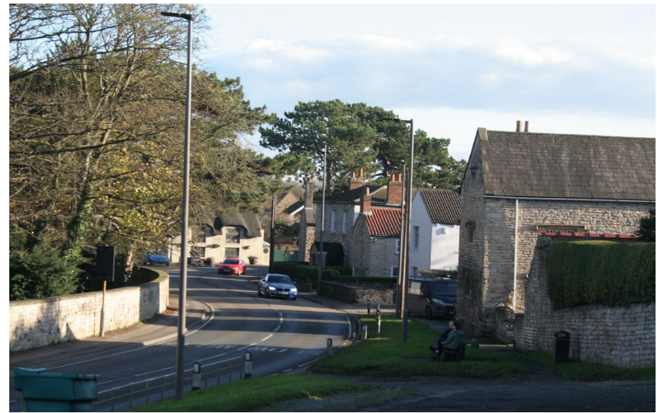
Townscape view 4, looking east down Main Street by St Wilfrid's churchyard
