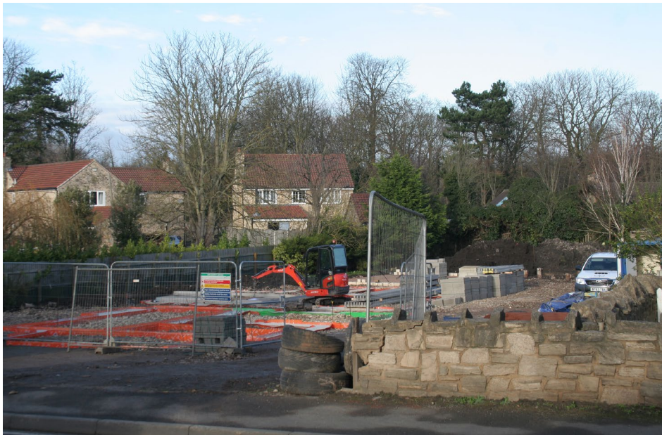
The foundations of an infill development in the grounds of 16 Main Street
