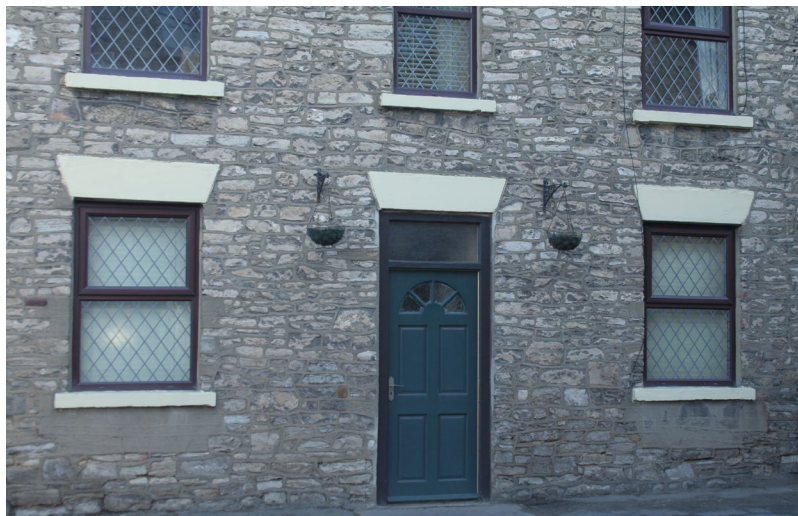
uPVC windows in brown on a traditional magnesien limestone property on Main Street
