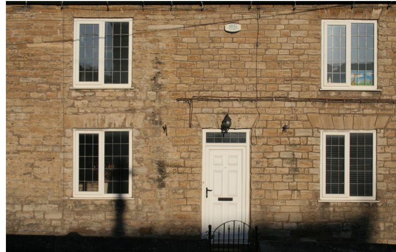
uPVC windows and door on a traditional magnesien limestone property on Main Street
