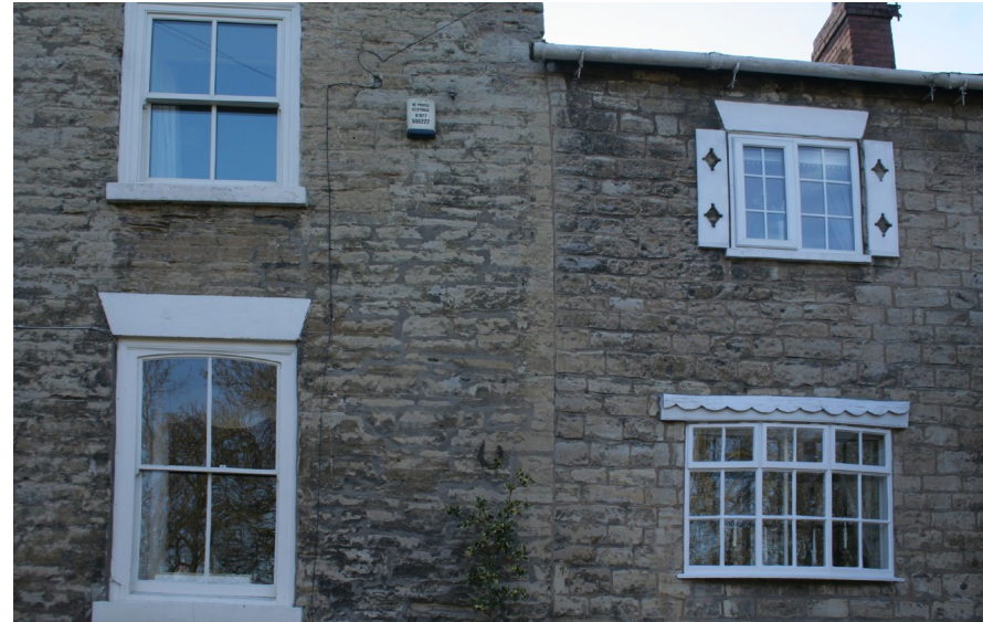
Timber sliding sashes on a traditional Magnesian limestone dwelling. Note the slight difference between the upper and lower sash. The upper is probably a recent replacement. Contrast this to the windows on the right.
