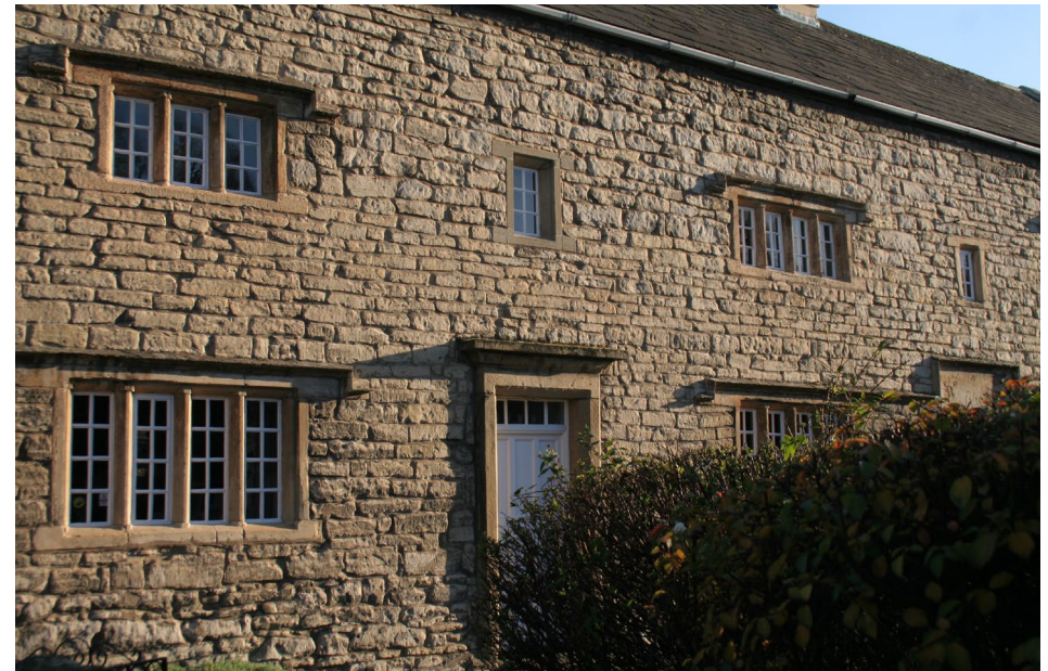
Magnesian limestone on the Grade II listed The Manor House in sunshine
