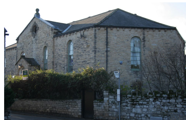
Welsh slate roof of the Grade II listed Methodist Church on Water Lane.
